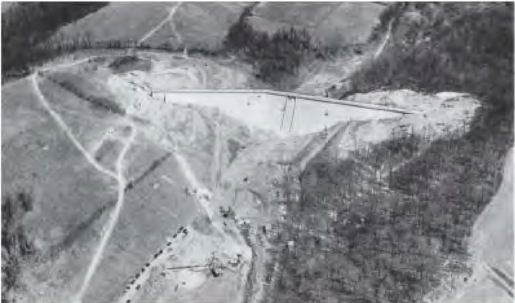
Hoopes Reservoir under construction, 1931.
